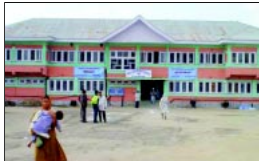
Figure 9.12: Retrofitted hospital building at Kupwara (Jammu and Kashmir, India)
