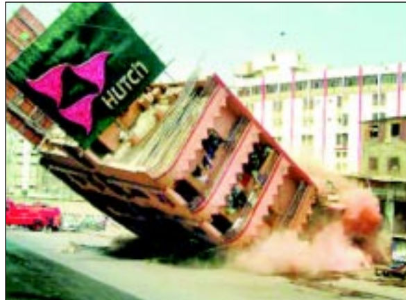
Figure 13.1: A building collapsed in Surat, India; however no casualty occurred as the fire brigade had evacuated the occupants in time.
