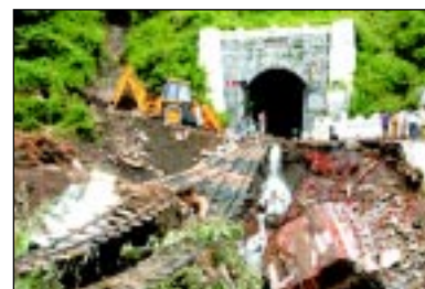
Figure 10.12: Damage to Koti railway station in Himachal Pradesh, India
