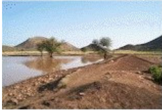
A Johad (water pond) constructed by the villagers
